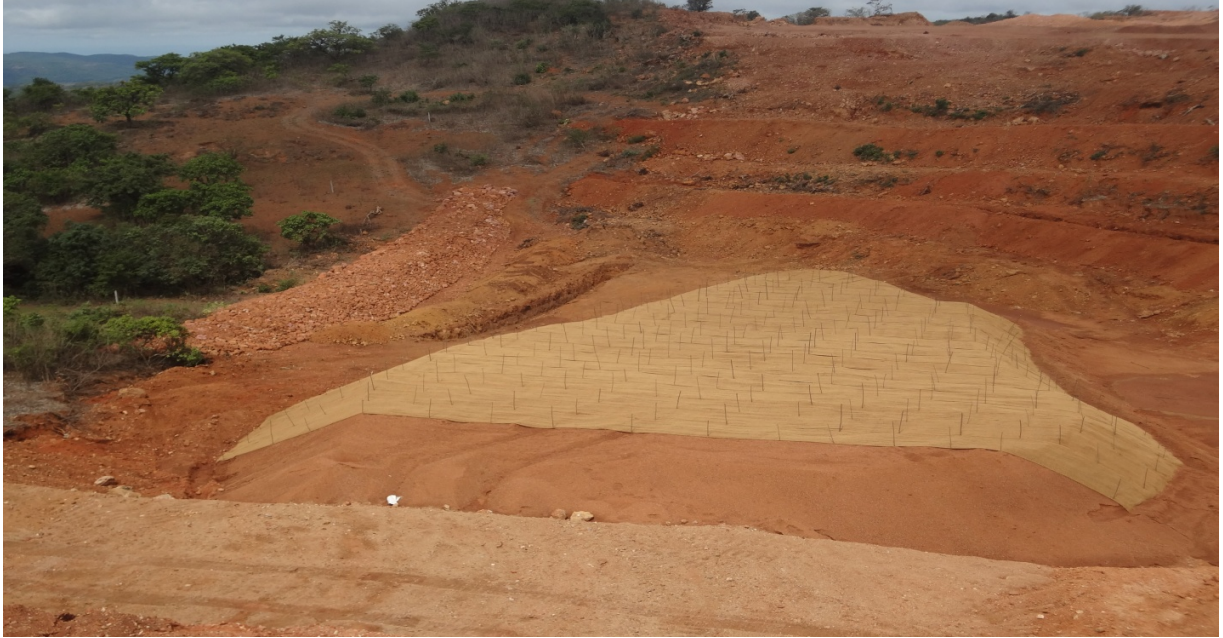
WASTE DUMP COVERED BY GEO TEXTILE BEFORE ON SET OF MONSOON
