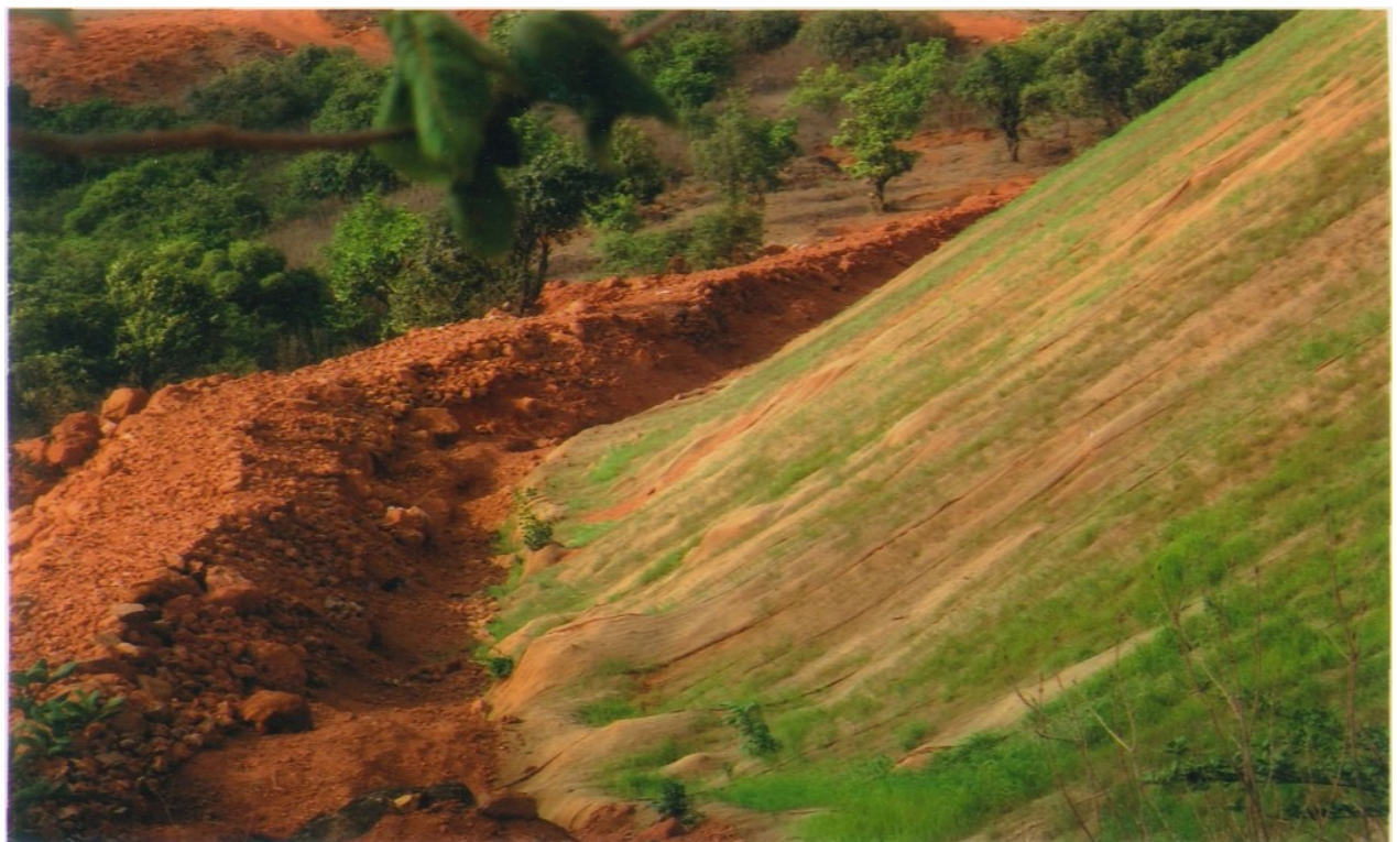
WASTE DUMP COVERED BY GEO TEXTILE DURING THE YEAR 2013-14
