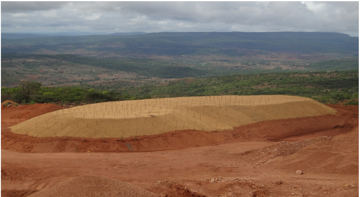
WASTE DUMP COVERED BY GEO TEXTILE BEFORE ON SET OF MONSOON
