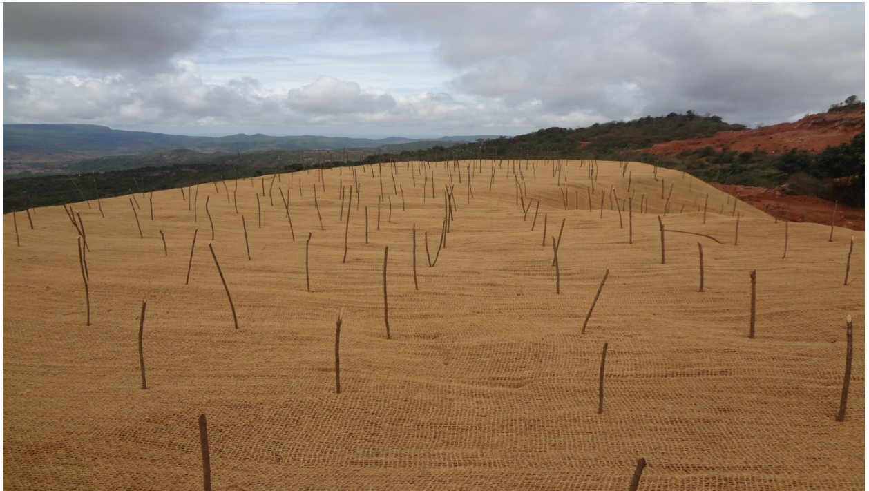
WASTE DUMP COVERED BY GEO TEXTILE BEFORE ON SET OF MONSOON
